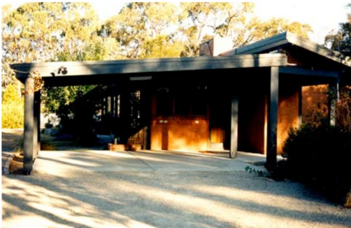
A mud-brick house with a passive solar design. There are no exposed windows on the west side of this house.
